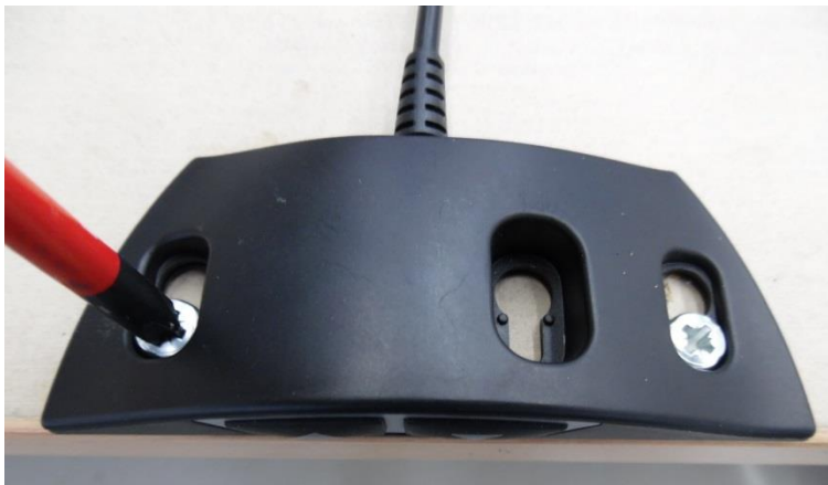
Figure 12 Attaching the simple manual switch UBM-F/2-p
